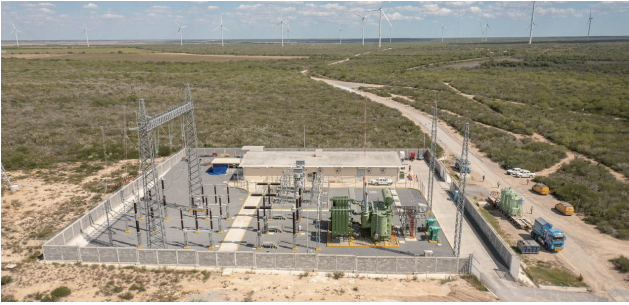
Mexico | Reynosa Wind Power Station 400kV 225MVA Power Transformer Project
