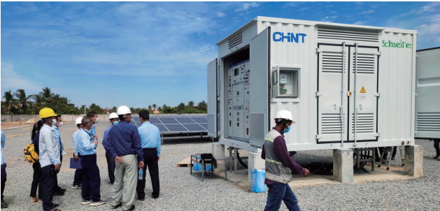
Cambodia | 1.8MW Ground PV EPC Project
