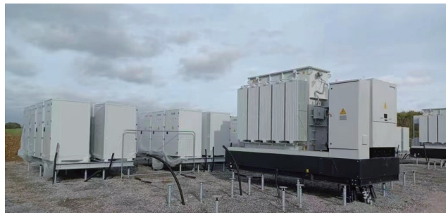
UK | 11-33kV Skids for Trina BESS Project
